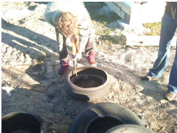
Figure 5 - Removal of side wall.
