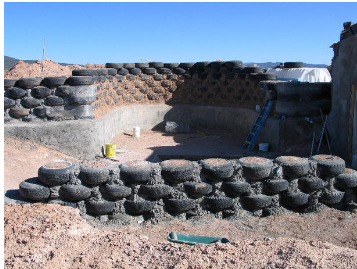
Figure 2 - Rammed Tire Structure during construction [13].
