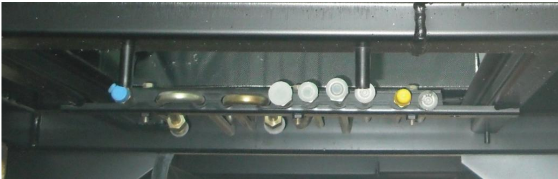
Figure 18 – Image of hydraulic bar from underneath cab
