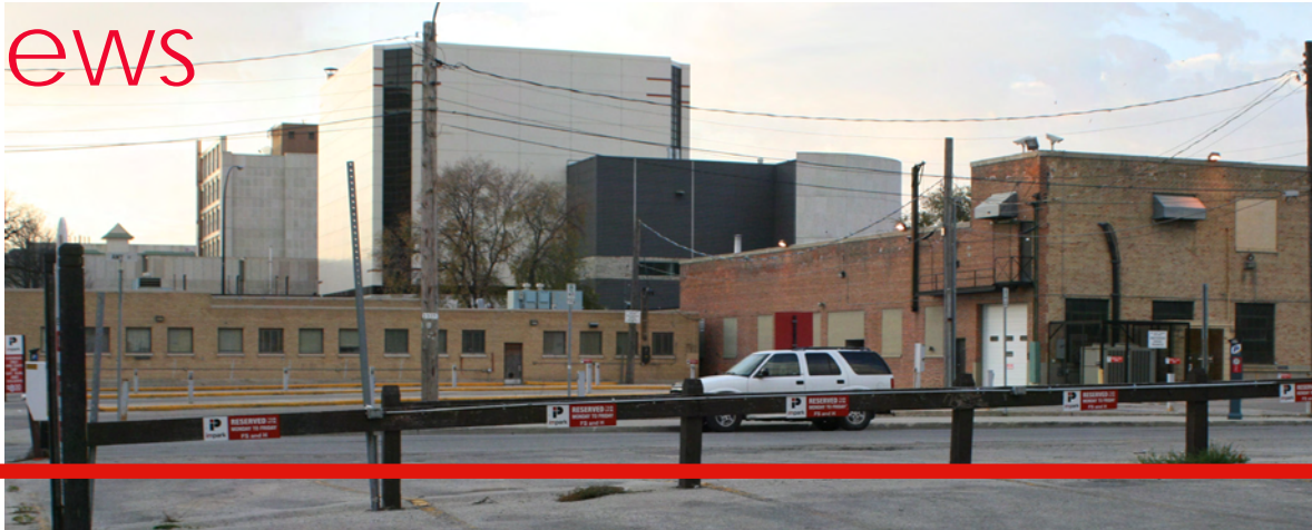
Figure 64 West view from James Avenue Pumping Station. Image by author.
