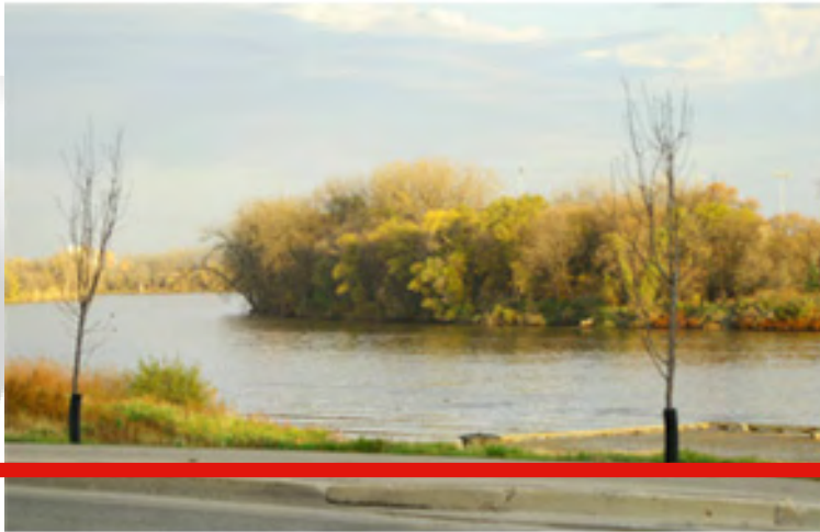
Figure 67 East View of James Avenue Pumping Station. Image by author.
