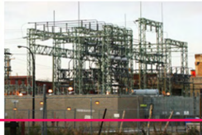
Figure 70 North View of James Avenue Pumping Station Image by author.
