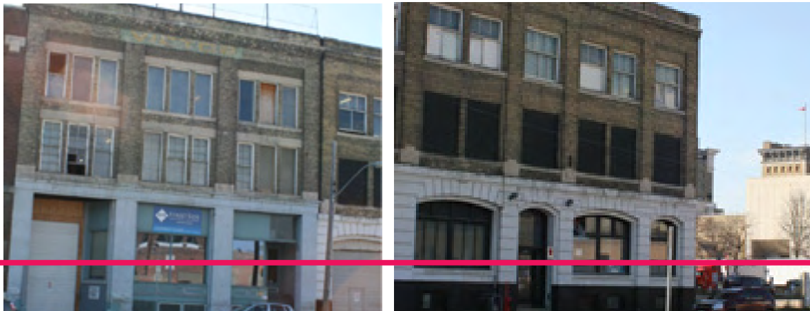
Figure 65 (right), Figure 66 (left) South View from James Avenue Pumping Station. Image by author.
