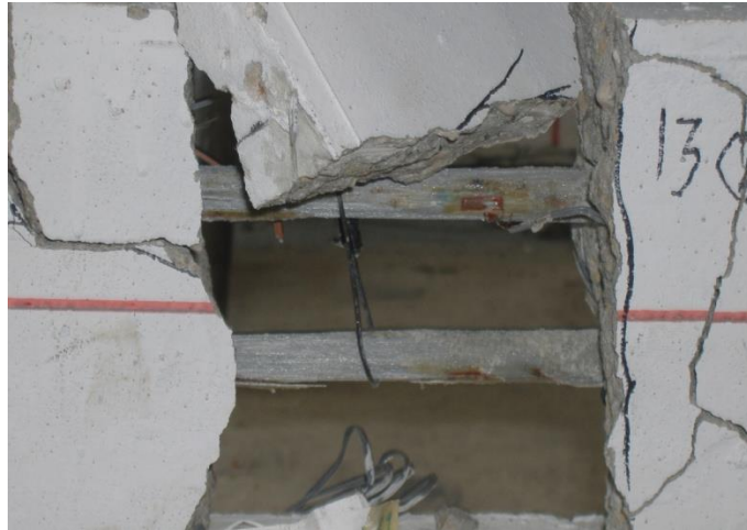
Figure 4.35 Failure Mode of Strap 35% III-A
