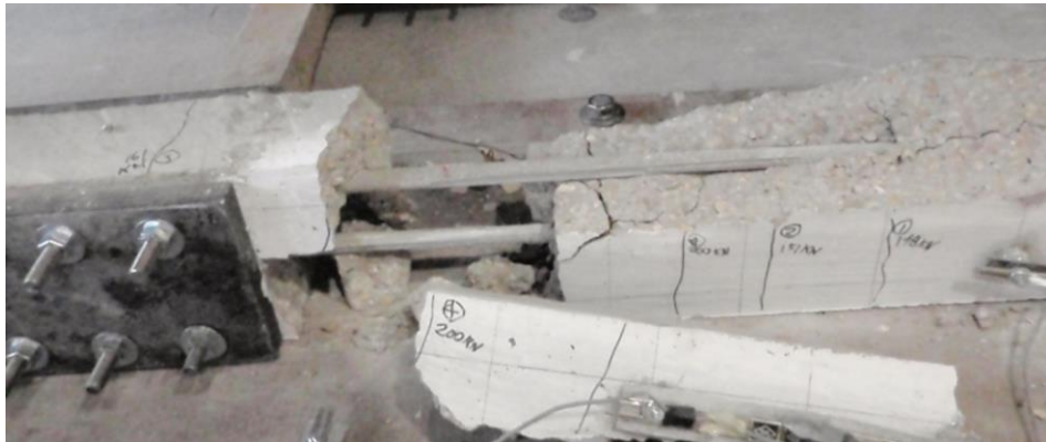
Figure 4.64 Failure Mode of Strap 45% III-B
