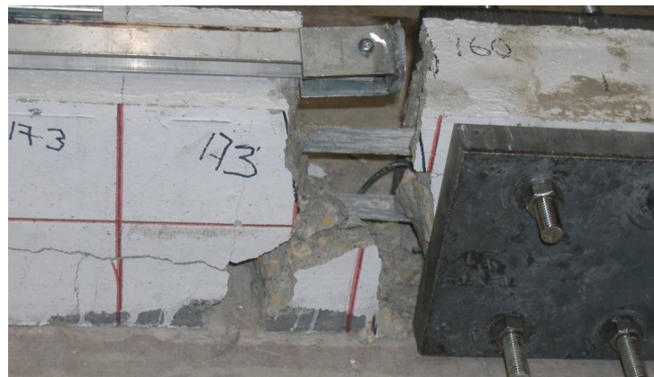
Figure 4.39 Failure Mode of Strap 45% II-A
