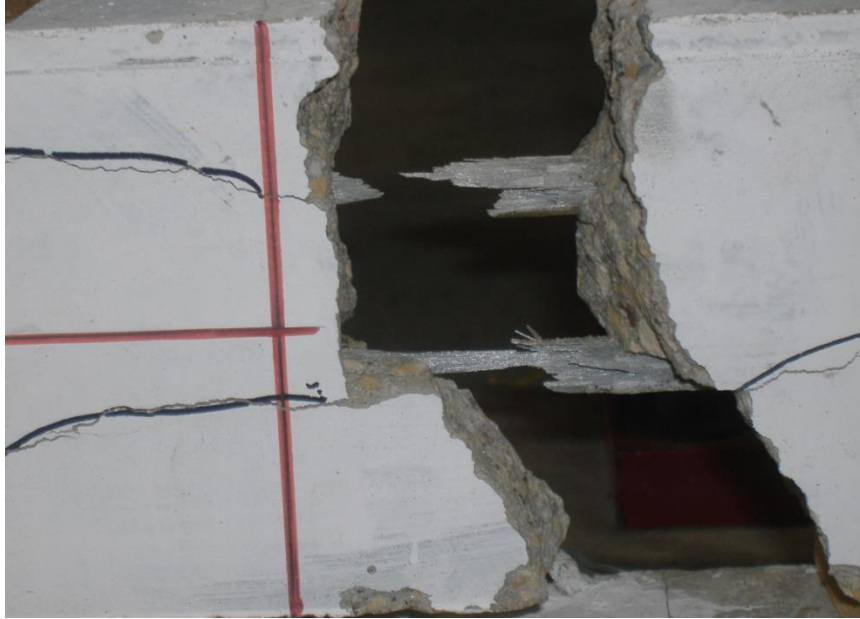
Figure 4.45 Failure Mode of Strap 55%III-A
