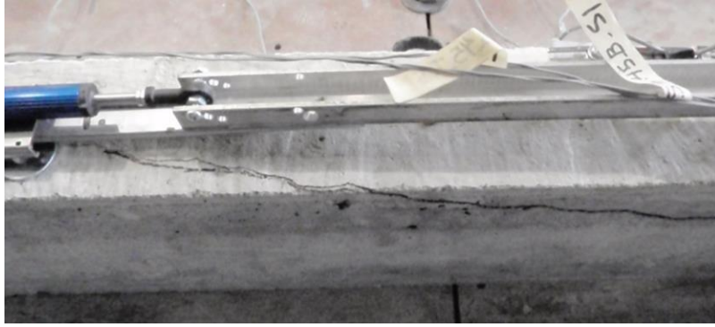
Figure 4.63 Horizontal Cracks on Strap 45% III-B
