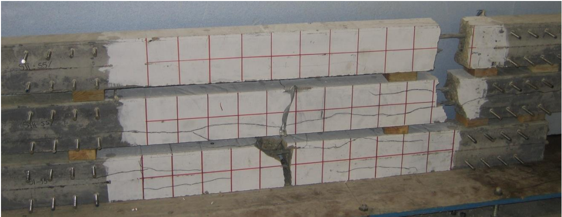
Figure 4.49 Crack Pattern and Mode of failure of Straps Prestressed at 55%-A
