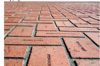
Figure 95 Bricks in Pioneer Courthouse Square Copyright uniquely-portland-oregon.com
