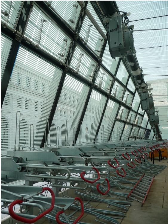
Figure 65 Interior View Copyright KPG Design Studio
