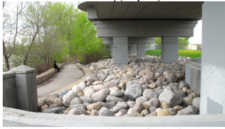
Figure 10 View southwest, from site
