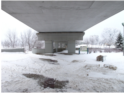
Figure 36 View southwest, from site
