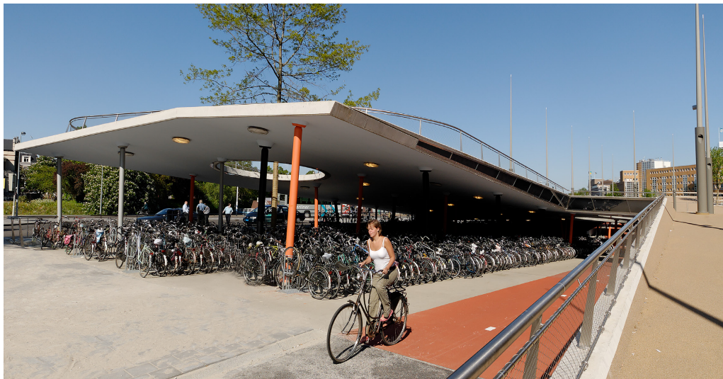
Figure 79 Entry to underground bike parking Copyright KCAP Architects & Planners
