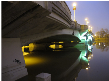
Figure 33 View of norwood bridge, from site
