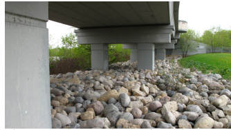
Figure 12 View southwest, from site
