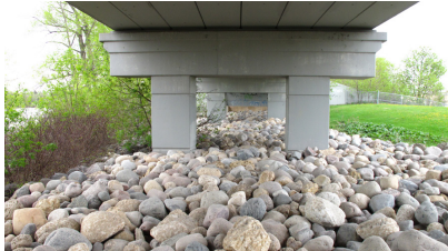
Figure 13 View southwest, from site
