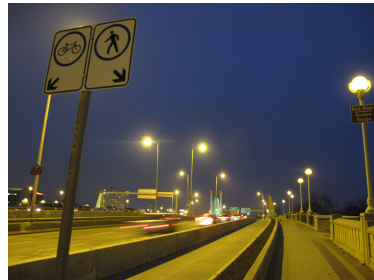
Figure 30 View of norwood bridge, from site
