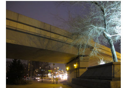
Figure 29 View north, toward site
