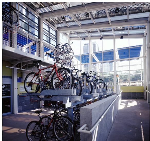
Figure 69 Interior bike storage Copyright Nathan Kirkman
