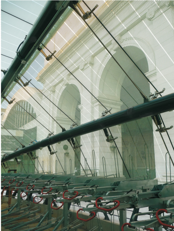
Figure 62 Interior View Copyright KPG Design Studio
