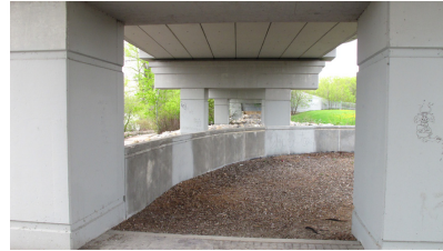
Figure 14 View southwest, from site
