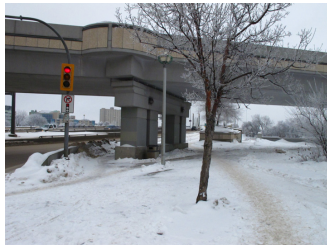
Figure 42 View southeast, toward site
