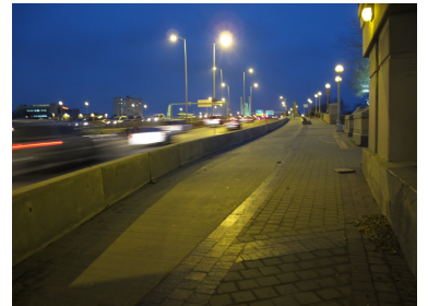
Figure 32 View of Norwood Bridge, from site
