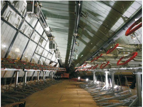
Figure 64 Interior View Copyright KPG Design Studio
