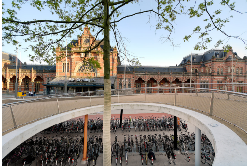
Figure 77 Groningen Central Station Copyright KCAP Architects & Planners
