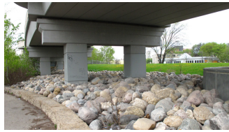
Figure 11 View southwest, from site
