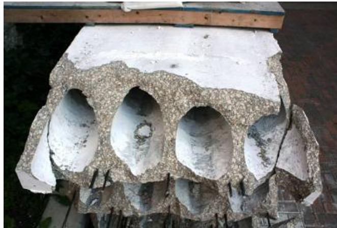
Figure G67: Failure Surface – End View (Web #5 on Far Right)
