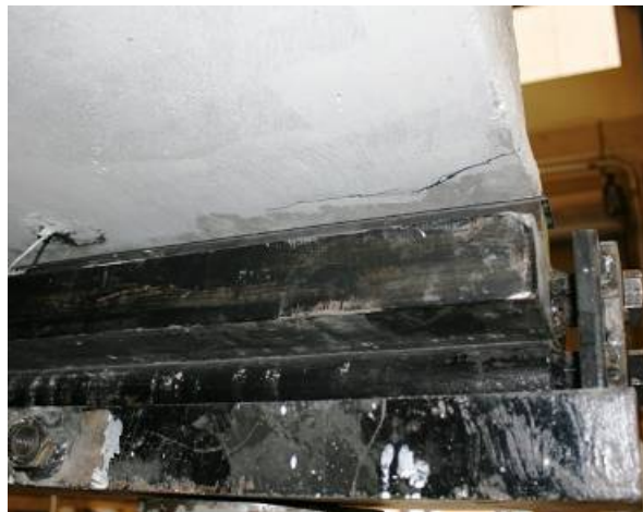
Figure G60: Cracking at Slab Underside – (Web #1 on Far Right)
