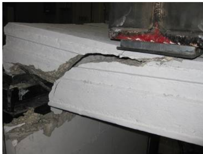
Figure G15: Web-Shear Cracks after Re-Loading Slab (Web #7 in Foreground)
