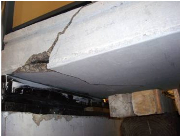
Figure G29: Transition from Flexural to Flexure-Shear Failure (Web #7 in Foreground)
