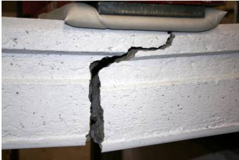
Figure G4: Initial Flexural Crack and Ruptured Strand at Web #1
