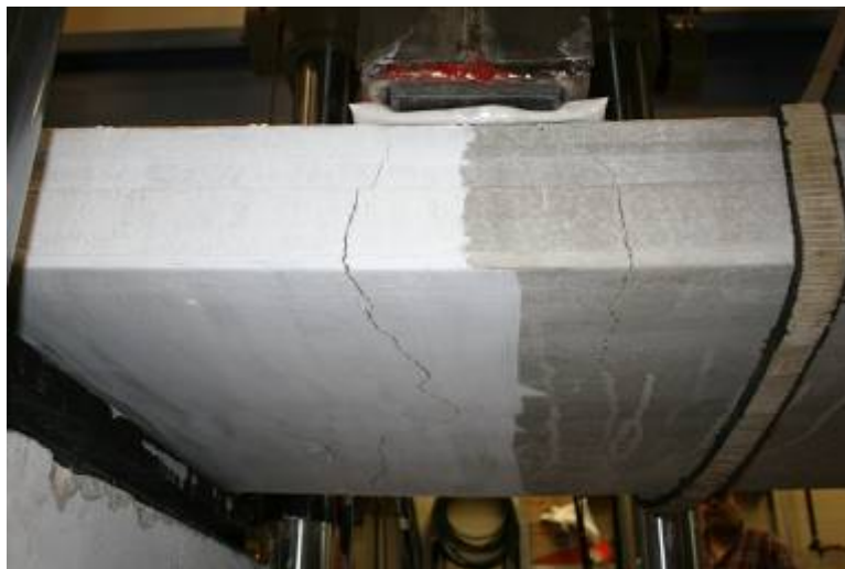
Figure G3: Underside of Slab at Web #7
