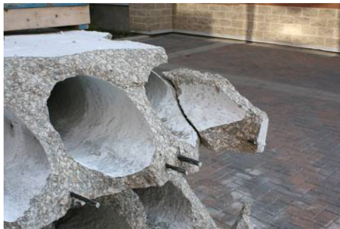
Figure G68: Failure Surface (Web #5 on Far Right)
