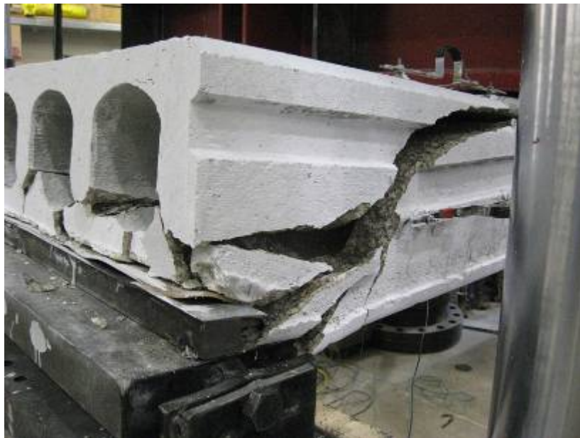
Figure G23: Web-Shear Cracks after Reloading (Web #7 in Foreground)
