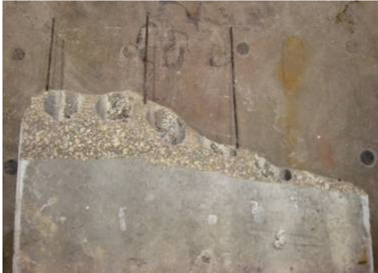
Figure G30: Failure Surface – Plan View (Web #1 and Ruptured Strand on Far Right)
