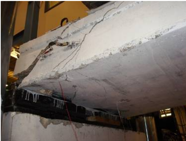
Figure G45: Underside of Slab at Web #7
