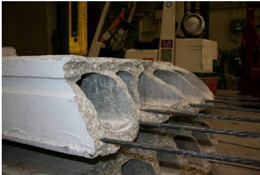
Figure G42: Failure Surface (Web #1 in Foreground)
