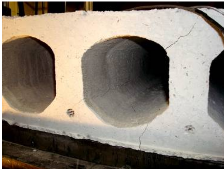
Figure G13: Additional Cracks in Webs #2 and #3 at (117 kN)
