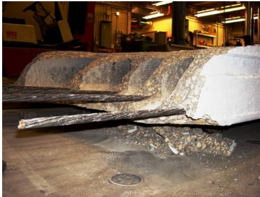
Figure G17: Failure Surface – Elevation View (Web #7 in Foreground)
