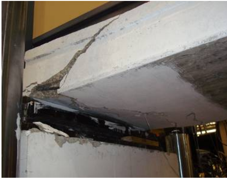
Figure G38: Transition to a Web-Shear Failure (Web #7 in Foreground)
