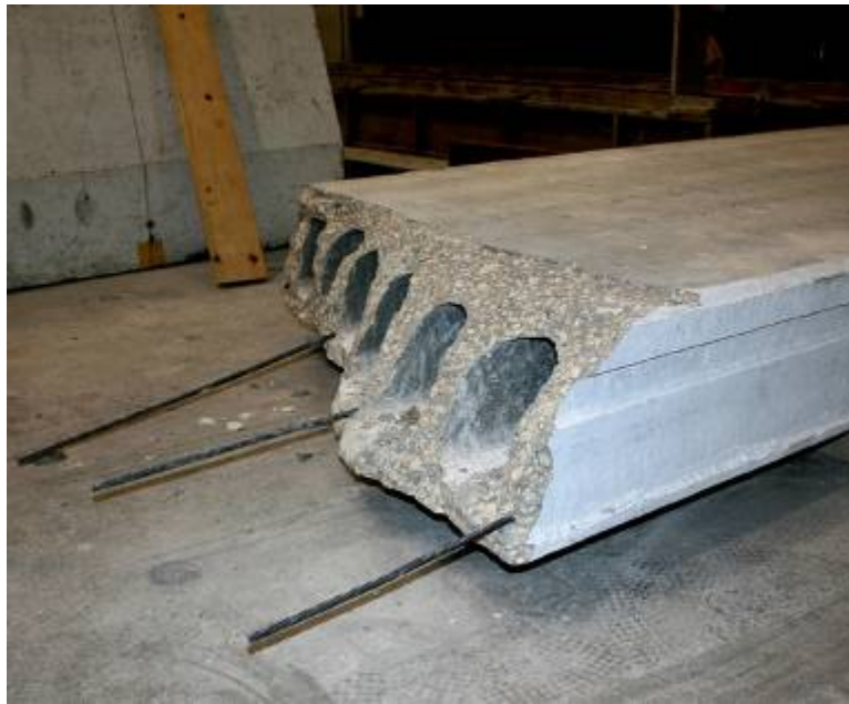
Figure G31: Failure Surface – Elevation View (Web #7 in Foreground)
