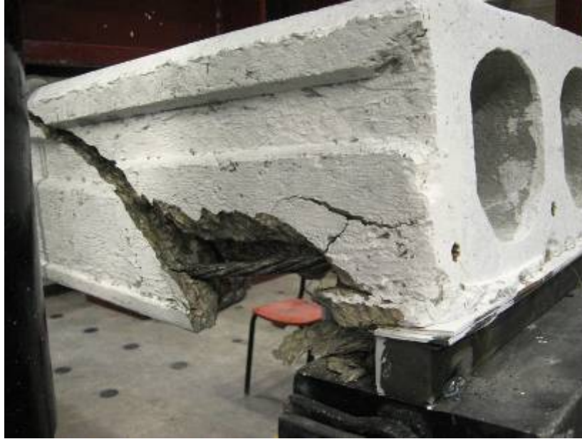
Figure G22: Web-Shear Cracks after Reloading (Web #1 in Foreground)
