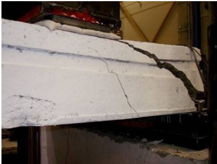
Figure G43: Initial and Secondary Web-Shear Cracks at Web #1
