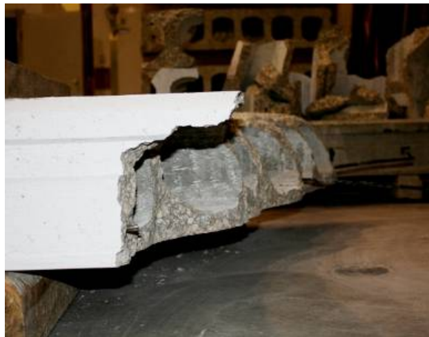
Figure G9: Failure Surface (Web #1 in Foreground)
