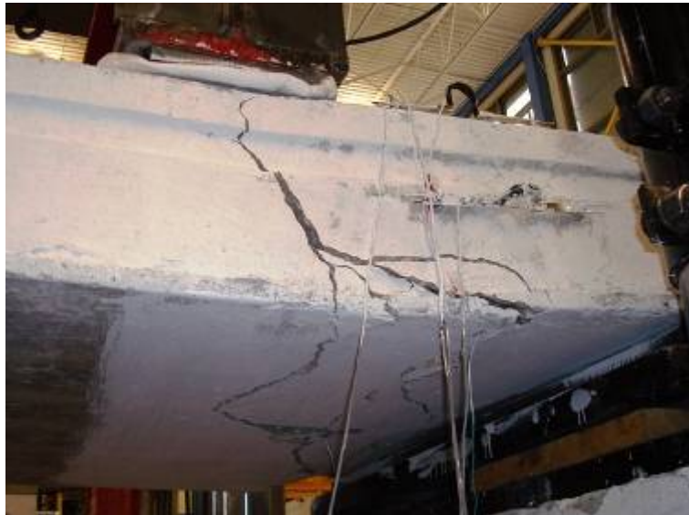
Figure G37: Diagonal Propagation of Crack across Slab Width
