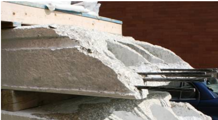
Figure G82: Failure Surface – Elevation View (Web #1 on Far Left)
