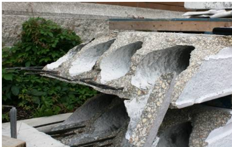
Figure G58: Failure Surface (Web #5 in Foreground)
