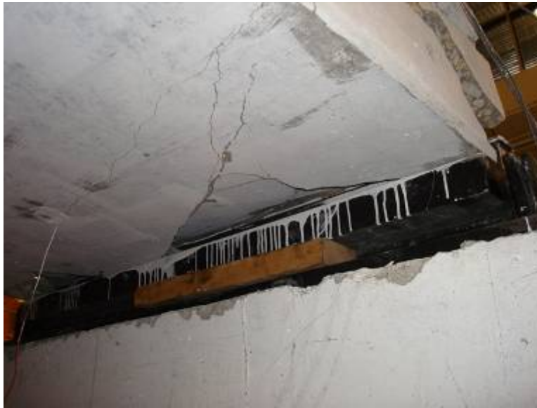
Figure G46: Underside of Slab at Web #1
