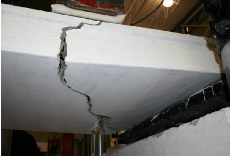
Figure G5: Diagonal Propagation of Crack across Slab Width (Web #1 in Foreground)
