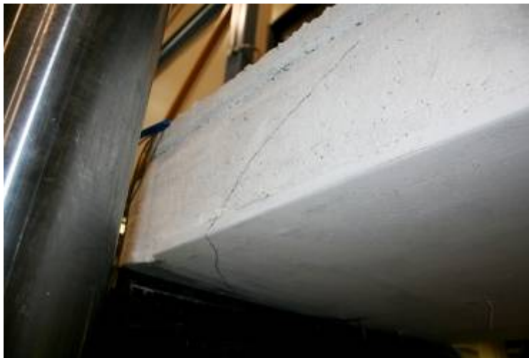
Figure G62: Cracking at Slab Underside – (Web #5 on Far Left)
