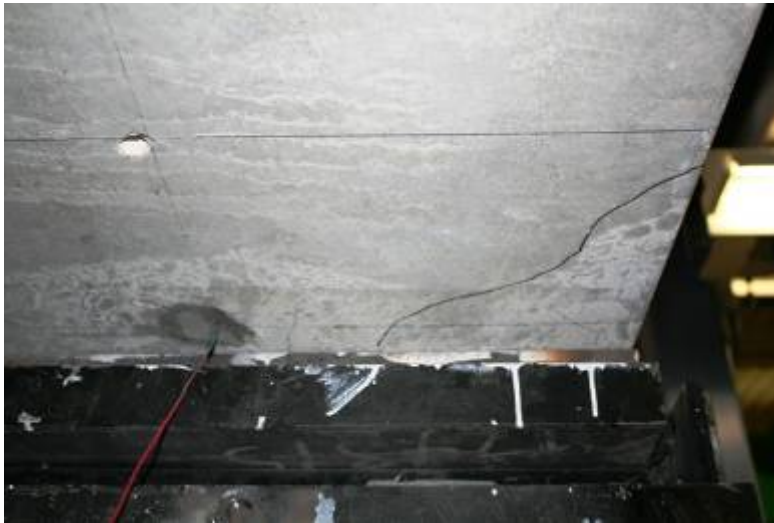
Figure G52: Diagonal Crack at Slab Underside (113 kN) – (Web #1 on Far Right)
