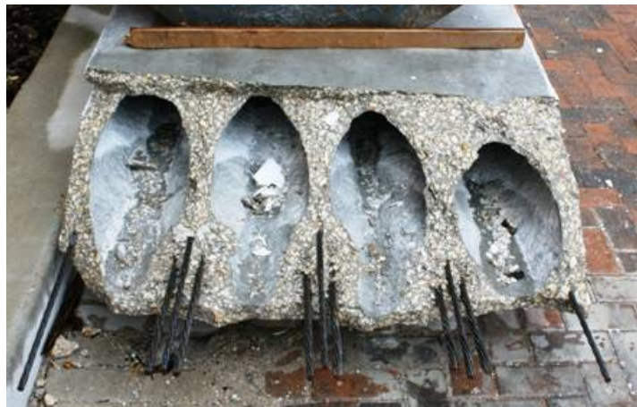
Figure G75: Failure Surface – End View (Web #1 on Far Left)
