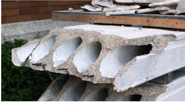
Figure G66: Failure Surface – Elevation View (Web #5 on Far Right)
