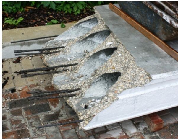
Figure G74: Failure Surface – Elevation View (Web #5 on Far Right)
