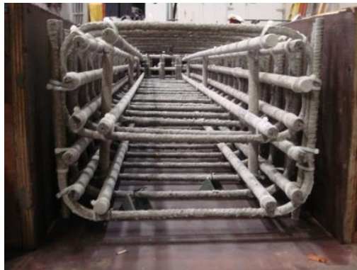
GG29-B11-J12 beam reinforcement
