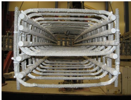
GG17-B11-J12 beam reinforcement
