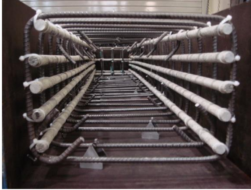
GS17-B11-J12 beam reinforcement
