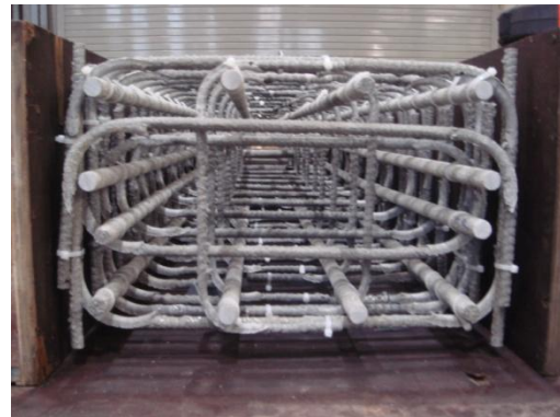
GG29-B11-J12 column reinforcement
