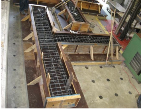
SS03-B06-J06 reinforcement cage
