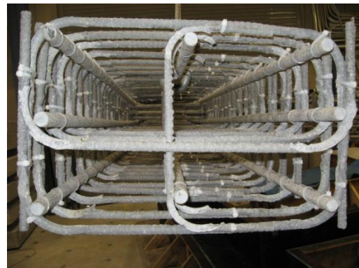
GG17-B11-J12 column reinforcement
