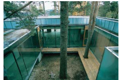
Fig. 4.31 (top): The reflective corrugated metal roof
