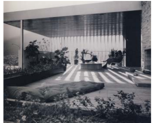
Fig. 3.4: The brise soleil system to provide shade on the terrace
