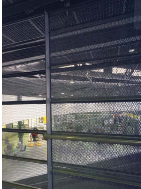
Fig. 4.35: View to lobby from upper level
