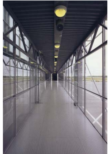
Fig. 4.33: Passage between terminal and airfield
