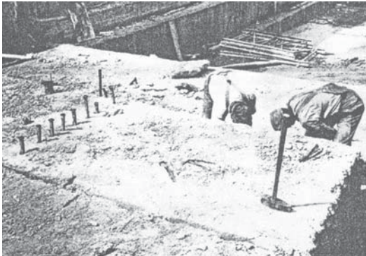
cutting of a mill block with plugs and feathers
