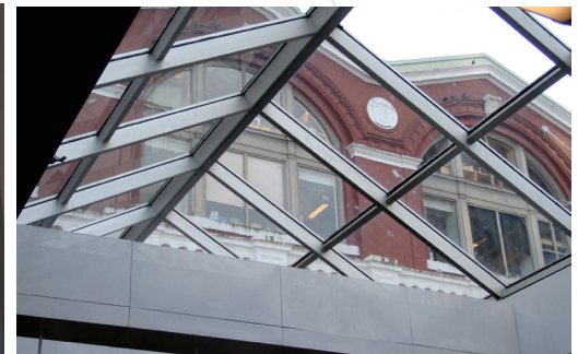
Figure 13: Skylights allow for as much natural light as possible
