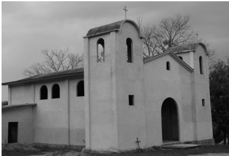
Plate 7.4: New church in San Martin Soyolapam, with construction part-financed by migrant contributions.
