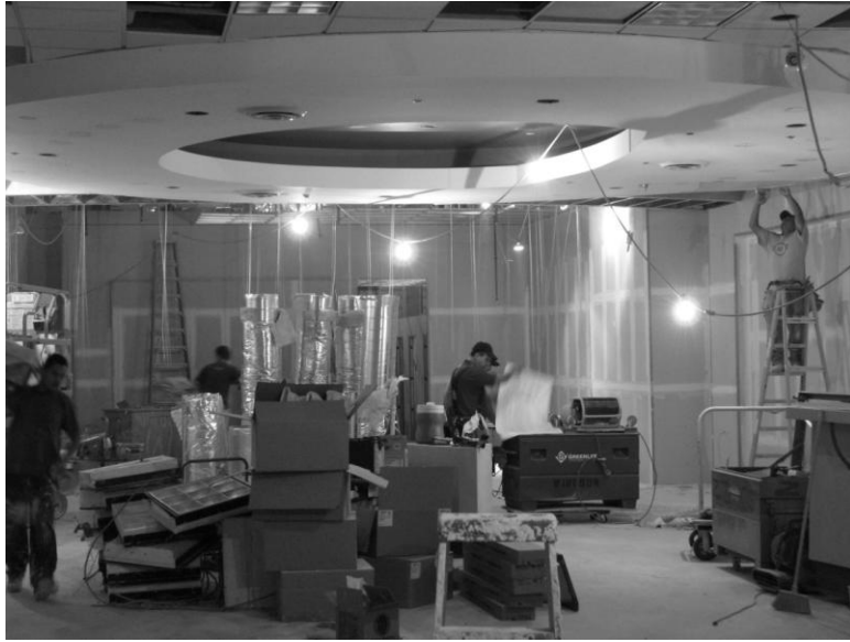
Plate 5.3: Migrant comaltepecanos working on store remodel in Glendale, CA Photo: Jim Robson
