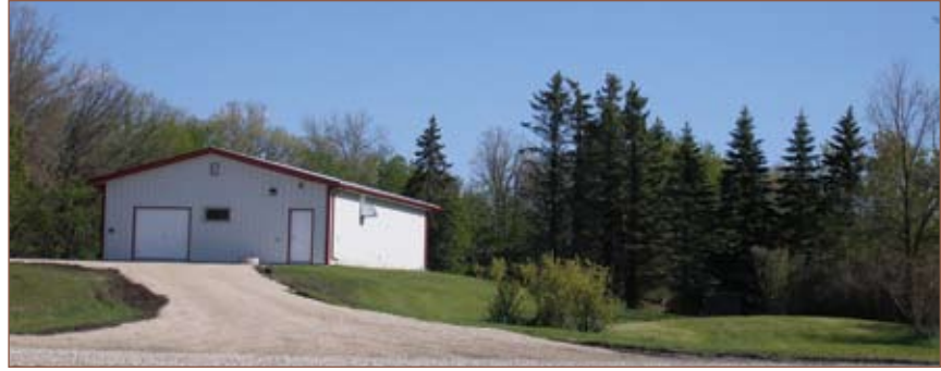
Figure 11: Waste water treatment facility.
