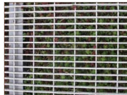
Figure 75: Metal grating serves as a covering for fragile groundcover allowing it to be used in a walkway.
