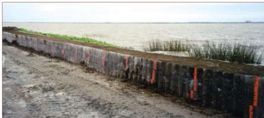
Figure 97: Geocell Rapid Deployment Flood Wall.
