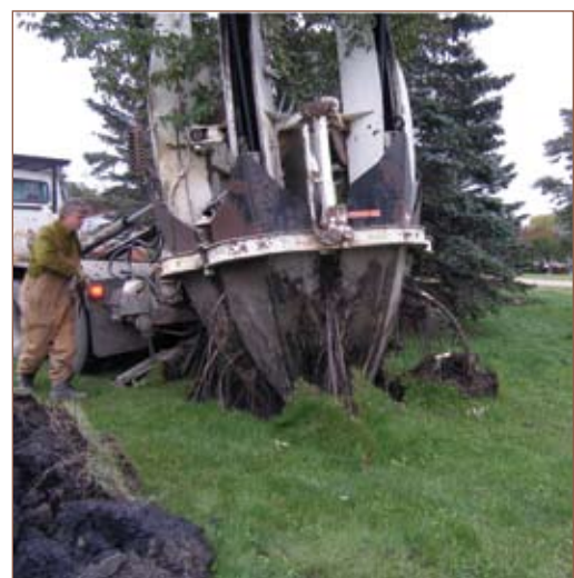
Figure 155: Beginning the lift.
