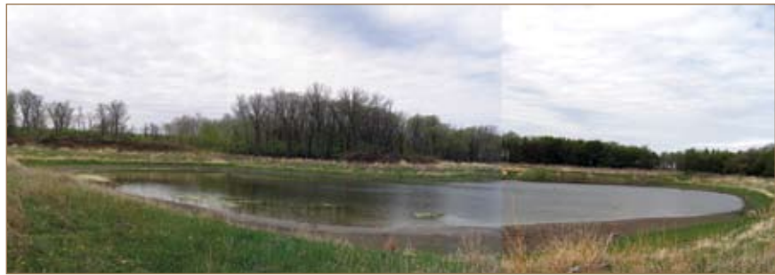
Figure 32: East external borrow pit.
