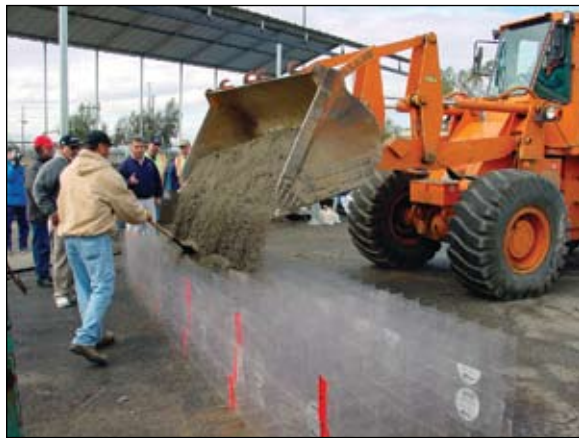
Figure 99: Geocell grids being filled.
