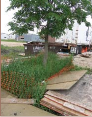
Figure 142: Mistreated elm. This elm was covered to mid-trunk level with dirt in 2008. In 2010, requirements to protect it during construction were ignored. It remains to be seen how long it will survive.
