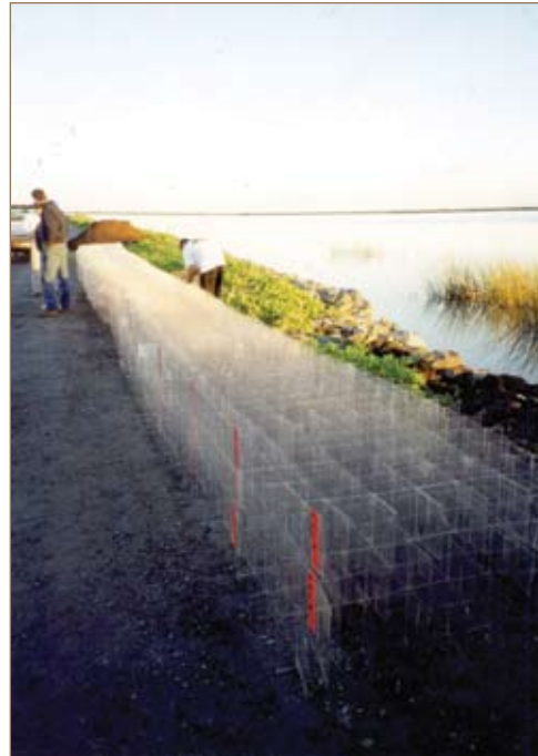
Figure 98: Geocell grids ready for filling.
