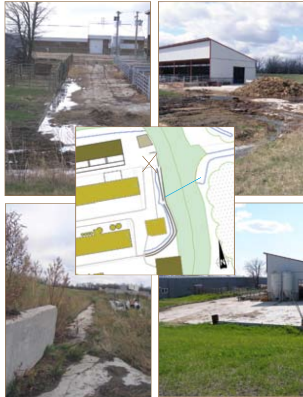
Figures 23: Cattle shed drainage. Upper left, clockwise: alley way draining, early spring; manure stockpile from cleaning sheds; area in summer; concrete drainage channel. Inset: location on site.
