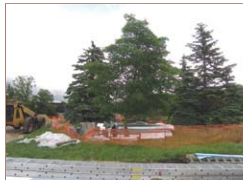
Figure 141: Construction material piled inside protective barrier. The contract required that the barrier be retained throughout construction.
