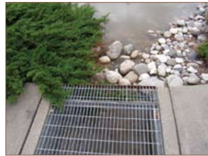
Figure 74: Metal grating serves as bridge.
