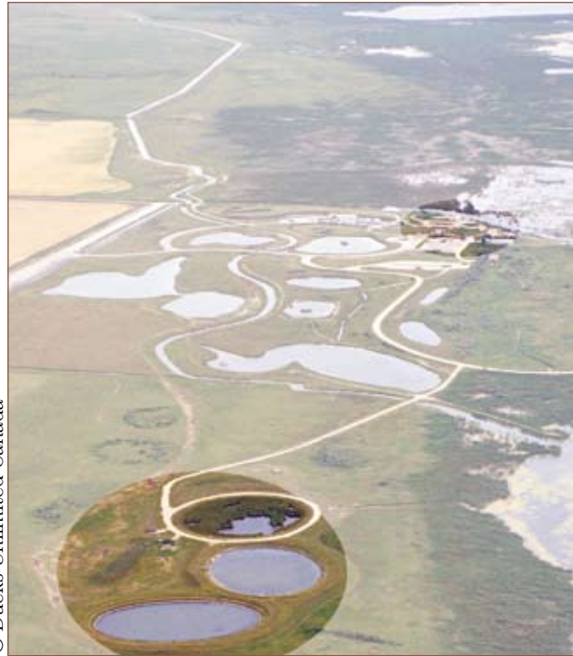
Figure 38: Ducks Unlimited Canada wetland wastewater treatment, Oak Hammock, Manitoba. The two bottom ponds are for settling solids; the upper is the treatment wetland.
