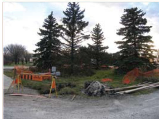
Figure 118: The foreground spruce needed to be removed due to root damage that occurred in 2008.
