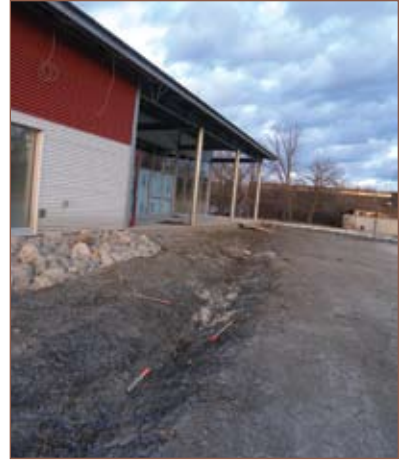
Figure 119: Drainage swale in front of the Discovery Centre designed to drain west.
