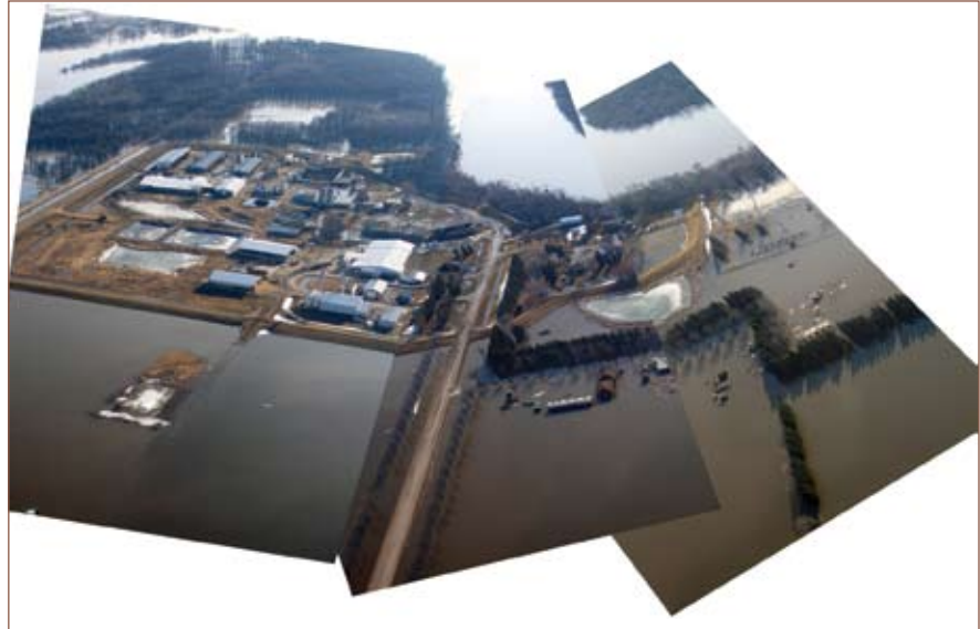
Figure 30: Water and the dike, spring flood 2009.
