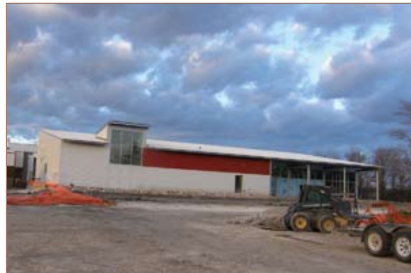
Figure 117: The Bruce D. Campbell Farm and Food Discovery Centre nearing completion, November 2010.
