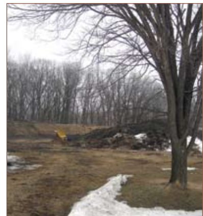
Figure 138: Proximity of excavated soil from wastewater treatment facility construction before tree protection was put in place.
