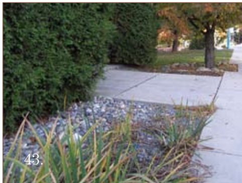
Figures 39 to 43: CK Choi Building wastewater treatment. 39. Inflow end of the C.K. Choi wetland, vegetation is more abundant due to the higher level of nutrients than at the outflow end, (43). 40. Basement composters for solid waste. 41. Vegetation mid-way. 42. Close-up of iris species and rhizomes. 43. End of treatment channel, clean water filters into the ground subsurface.
