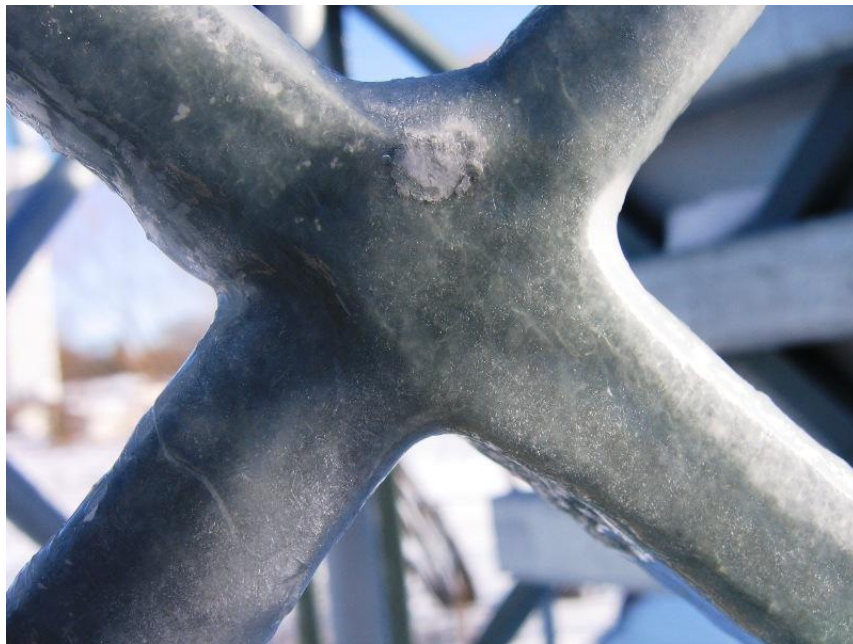
Figure 3.17: Ice on the diagonal bracing of FRP tower
