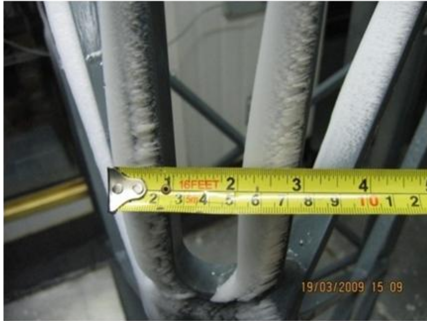
(a) Measured thickness of the hard rime ice
