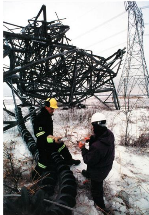
Figure 1.3: Hydro-Quebec pylon collapsed under the weight of the ice, near Drummondville, Quebec, January 1998 (Abley, 1998)
