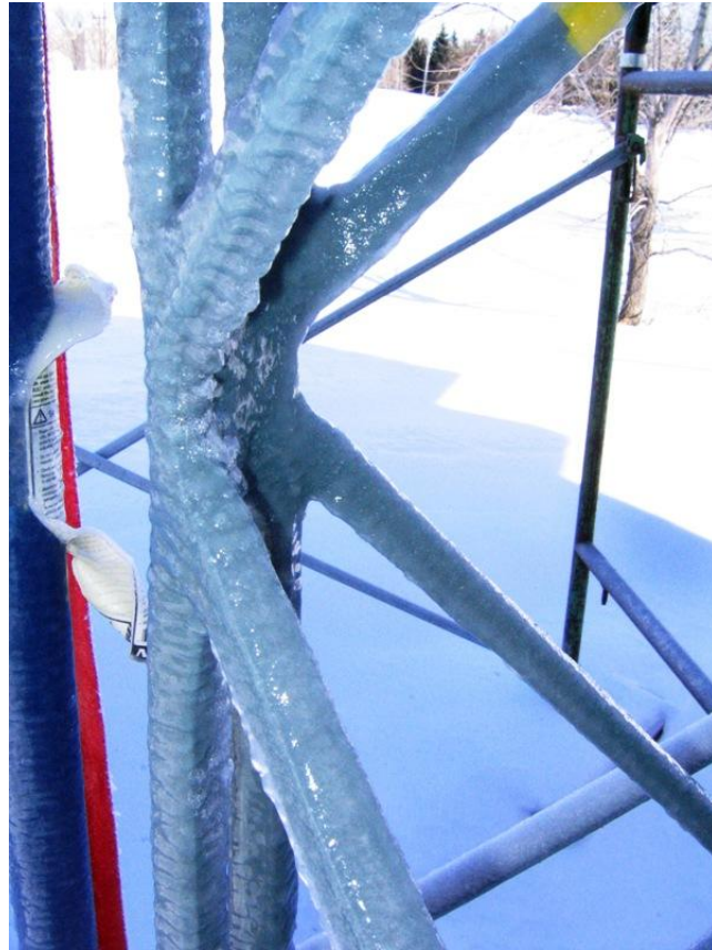
Figure 3.16: Iced chord of the FRP tower
