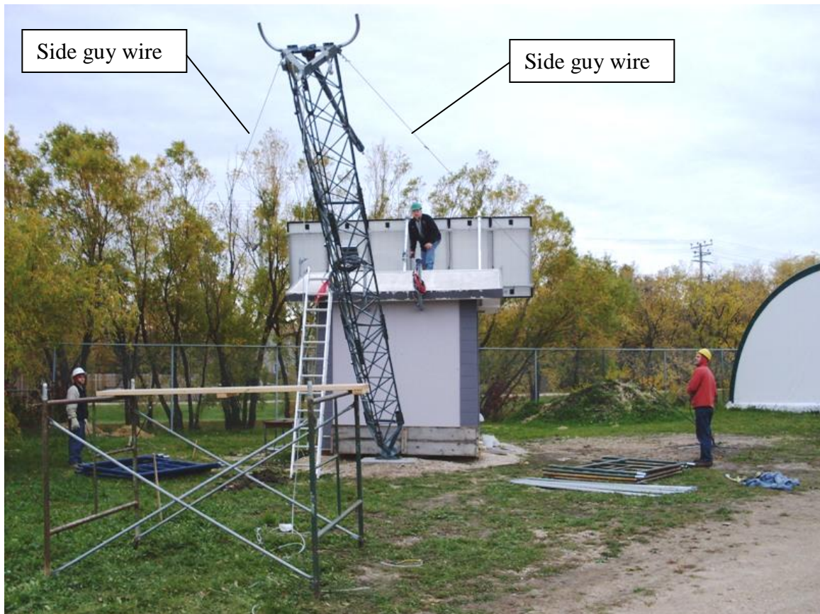
Figure 3.11: Erection of the tower
