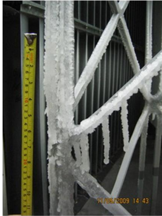
(a) Appearance of the glaze ice on FRP section
