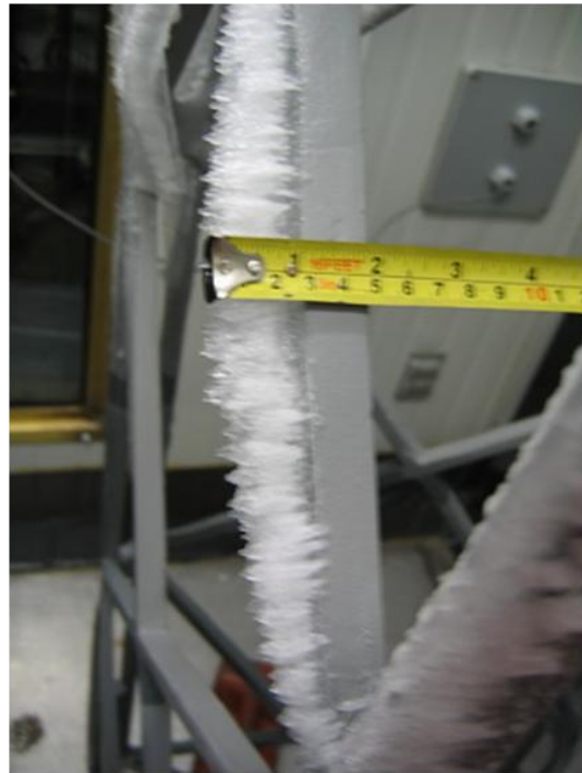
(b) Measured thickness of the glaze ice on the FRP section
