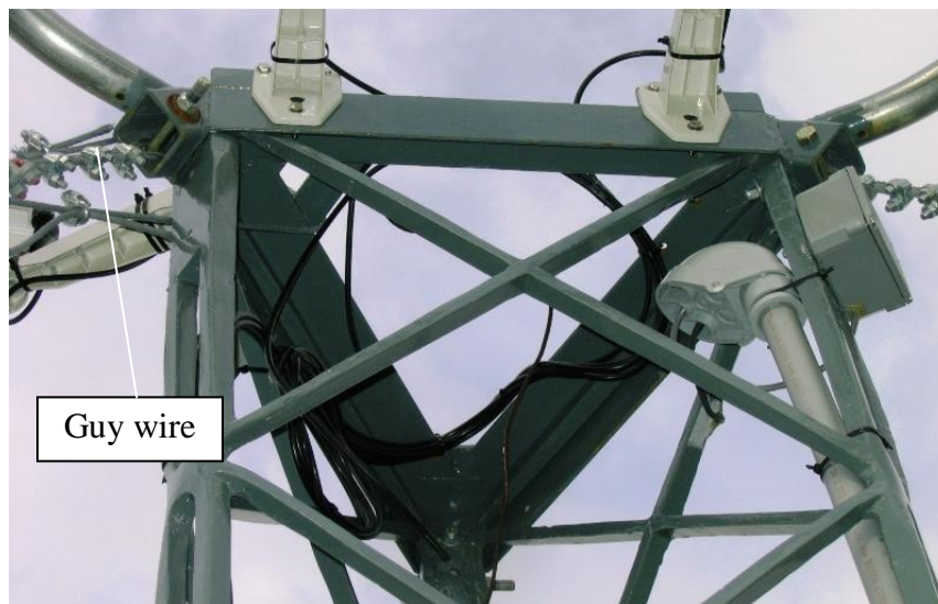
Figure 3.9: Guy wire attachment bracket
