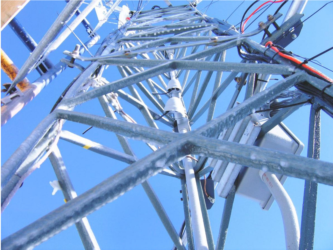
Figure 3.18: Iced members of FRP tower
