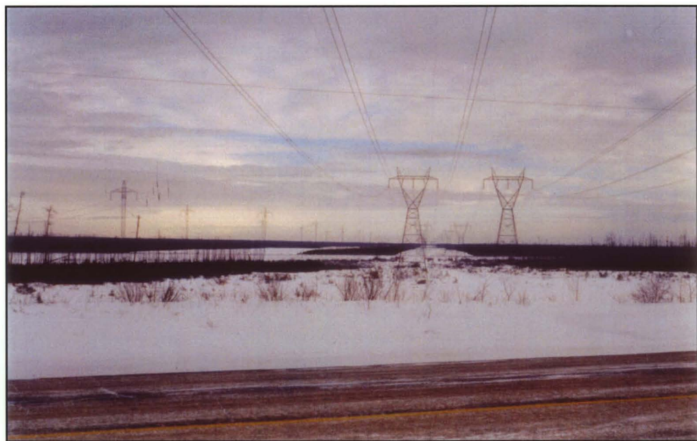
Plate 5: Hydro-electric transmission lines along Highway #6 north of Grand Rapids.
