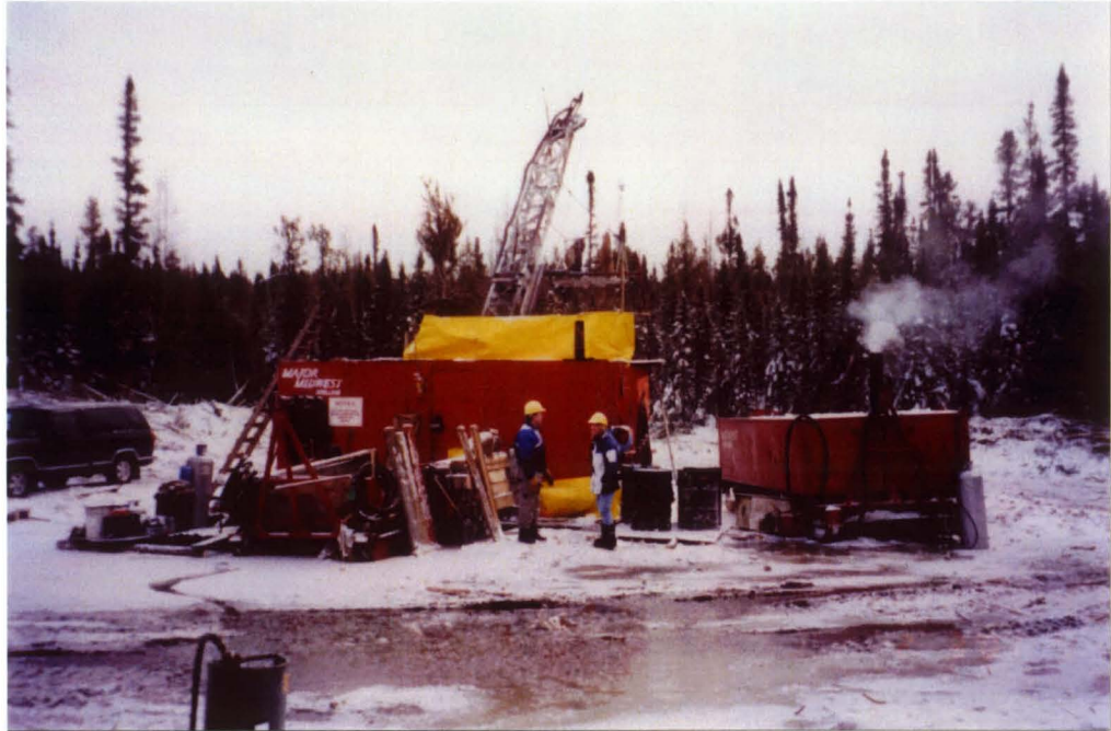
Plate 6: Drill site of Falconbridge Inc. located near William Lake.
