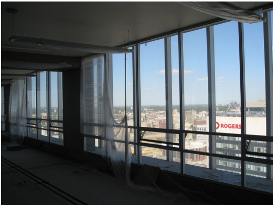
Figure 44. View from south of building looking northeast.
