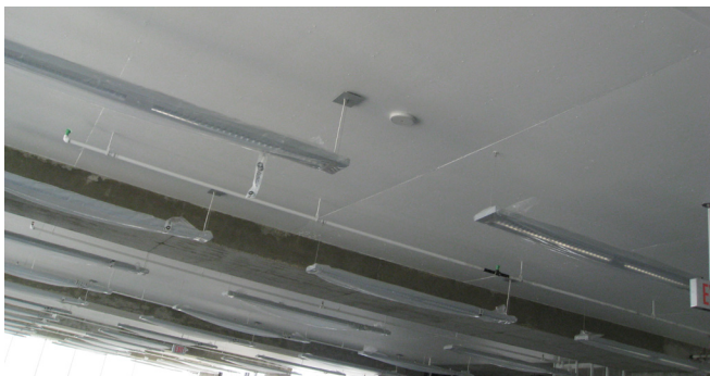
Figure 29. Concrete ceiling beams.
