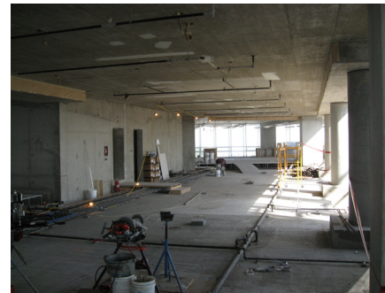
Figure 28. View on south side of the building looking east
