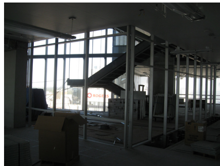
Figure 26. View of north atrium looking northeast
