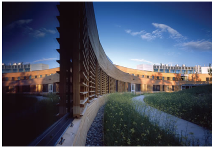
Figure 5. Exterior view of the front of the building.
