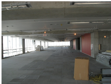
Figure 25. View of east side of building looking south
