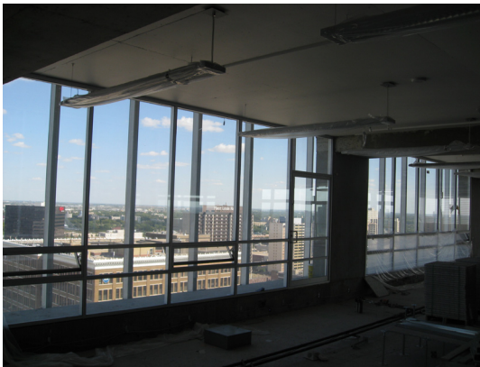
Figure 45. View from south of building looking southeast.
