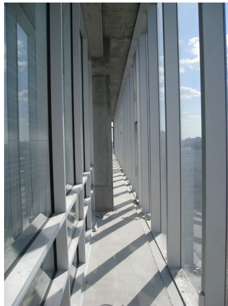
Figure 30. Double glass facade on west side of building.
