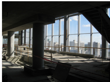
Figure 27. View of south atrium looking southeast
