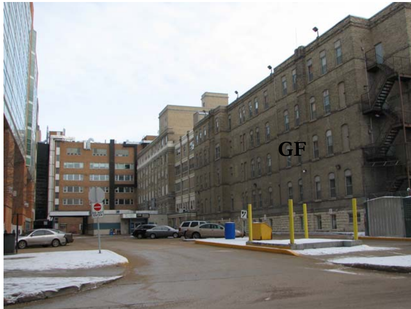
Figure 40. Adjacent parking and Site (located on the right). Used with permission by Health Sciences Centre Winnipeg
