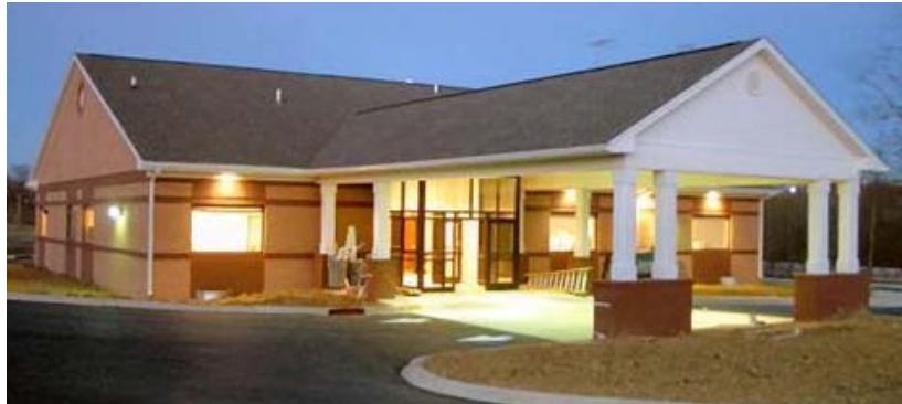
Figure 13. DaVita Dialysis Clinic in La Grange, Kentucky. Used with permission from Whitley Manufacturing Co. Inc.
