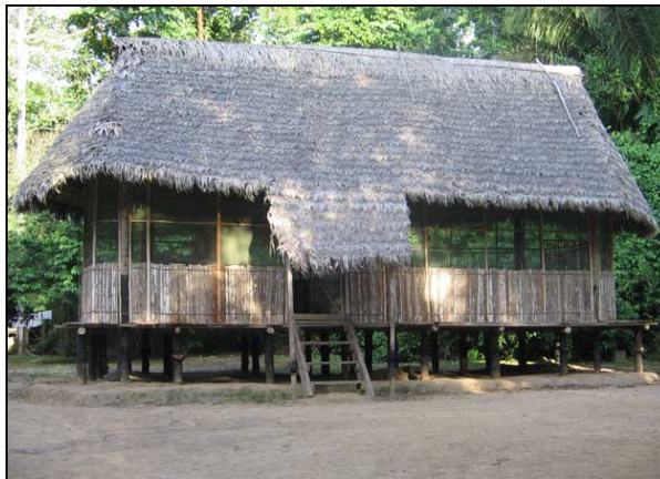
Figure 6: A Casa Matsigenka lodge building.
