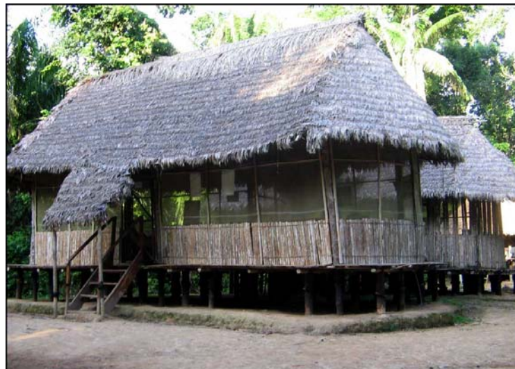
Figure 9: A Casa Matsigenka lodge building.
