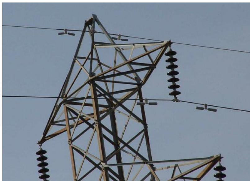
Figure 2.1: Photograph of skywire (top) and conductor (below)
