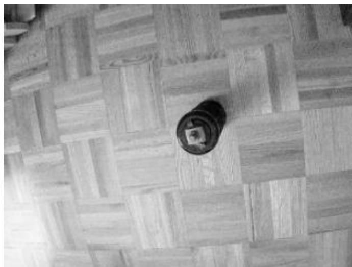
Figure 6.17: Line crawler view of the target insulator
