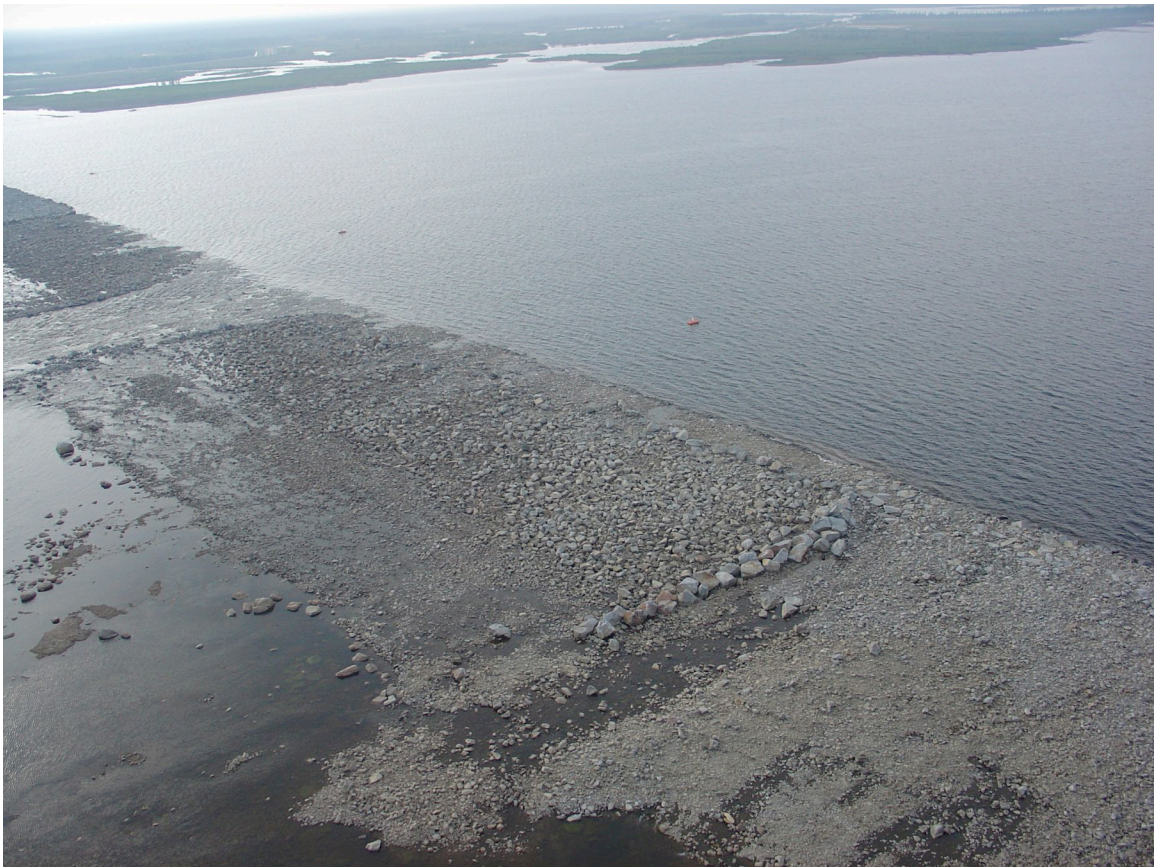
Figure 6. The lower Churchill River Weir (photo credit: used with permission from Warren Bernhardt, March 20, 2007)
