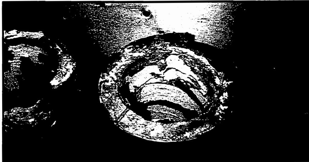
Figure 4.12(b): Top View of 300 mm Diameter Piles with Single Layer of GFRP Wrap After Failure
