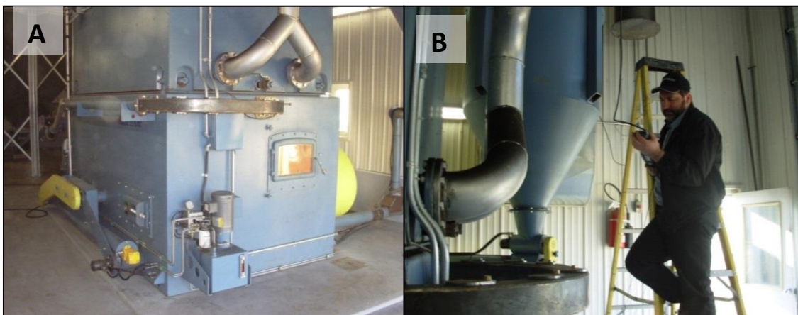
Figure 5.12. A) Blue Flame Stoker burner at the Sturgeon Creek Hutterite Colony burning densified cattail cubes; B) emission testing during cattail cube burn.
