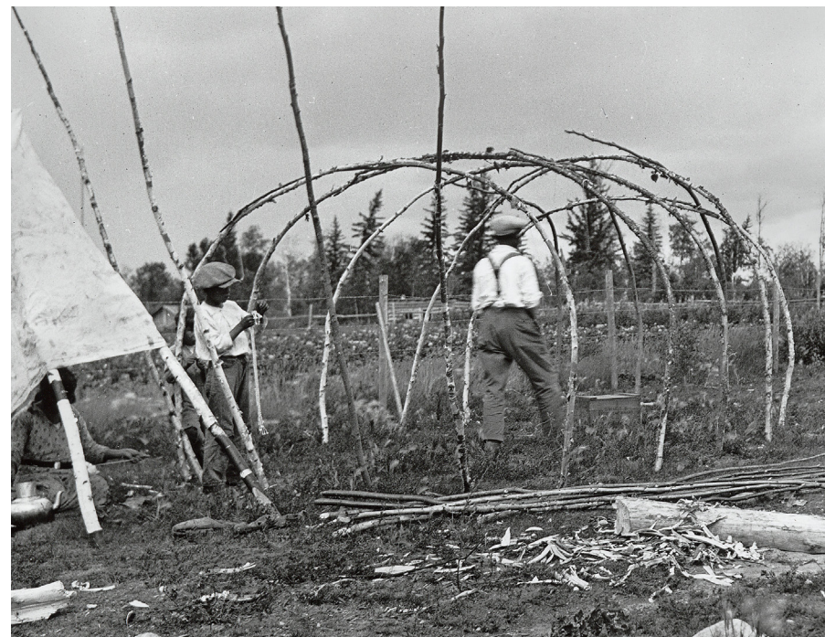
Figure 3.1.1.2 Working on Waginogan Framework Photograph by S. Boggs
