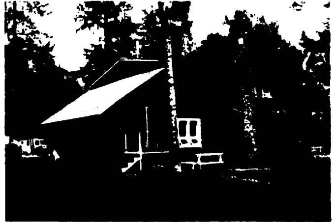
Fig. 64 The Research Centre (showing 1952 addition) (Photo by J. Wagner)
