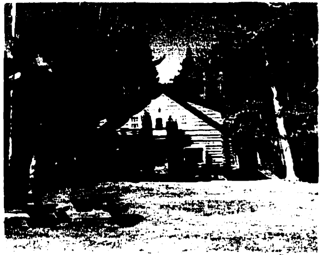
Fig. 70 View towards the Saddle Shed (Photo by J. Wagner)
