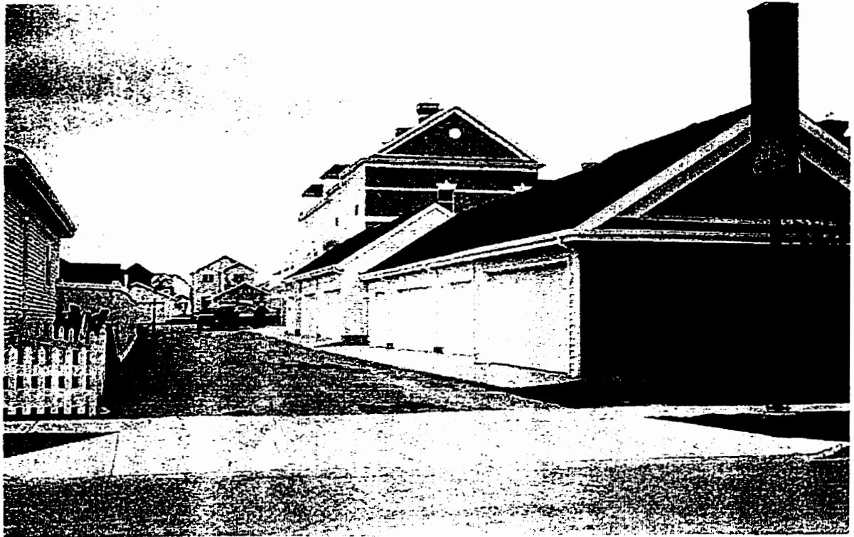
Figure 11 Garages are accessed from back lanes. Photo by author.
