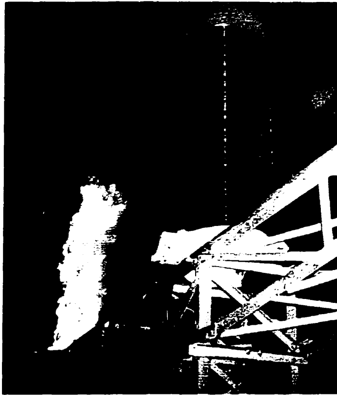
Fig. 1.2 Catastrophic failure of V13F due to ferroresonance.
