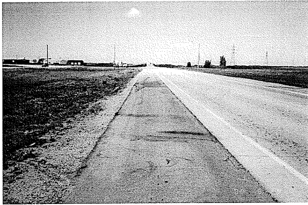
Perimeter Highway and Gunn Road
