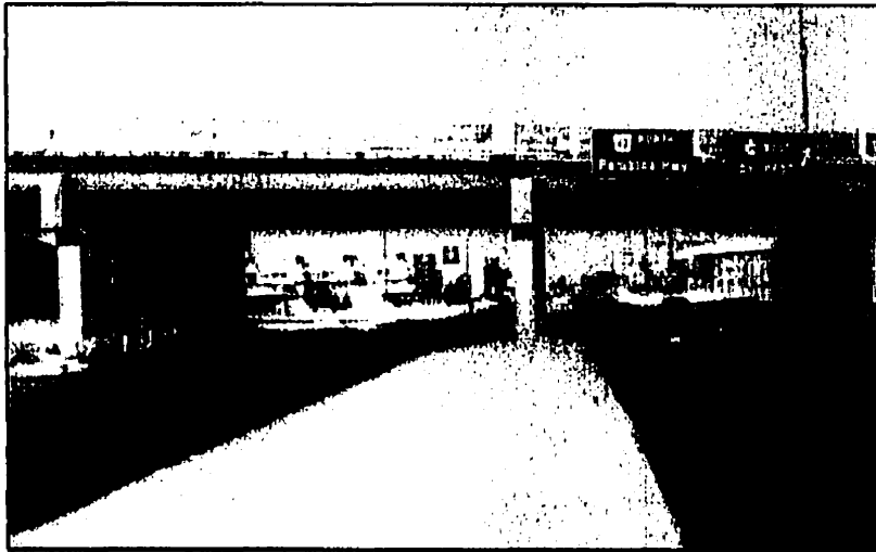
I-4 Pembina Highway at the Perimeter (photo F. Cholakis)
