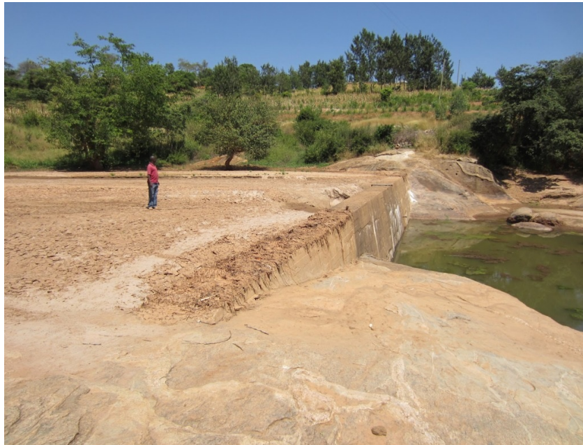
Photo 4.2: Sand dam built with Utooni Development in Kola (Wiens and Wiens 2012)
