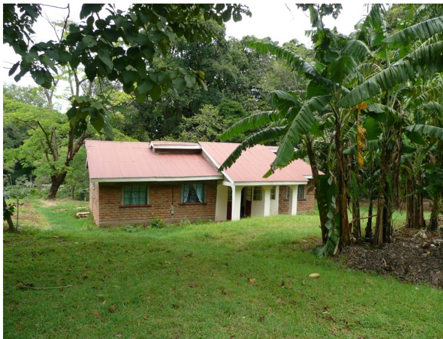
Photo 5.9: RSP guest house
