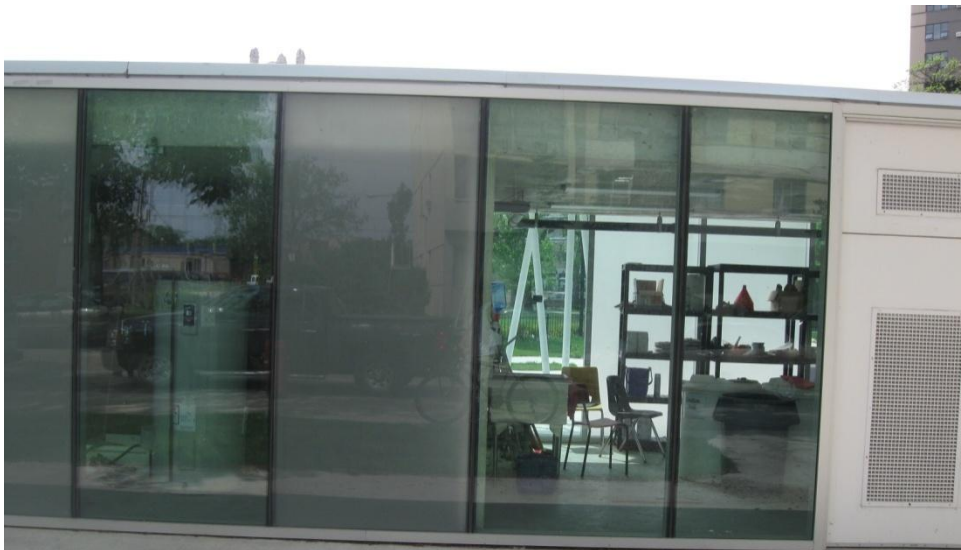
Figure 9. Maintenance Building. The building in the North side of the park is a see-through structure that provides park users with bathrooms, change rooms and also allows seeing the system powering the splash pad.
