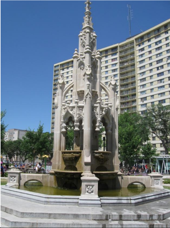
Figure 5. Waddell Fountain. The fountain was repaired as part of the rejuvenation of Central Park.
