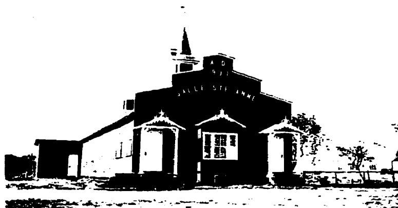
Figure 31: The Parish Hall was built in 1937 and was at one time used as a sewing factory. It was demolished sometime in the 1980s. (Photo courtesy Redemptorist Archives, Quebec)
